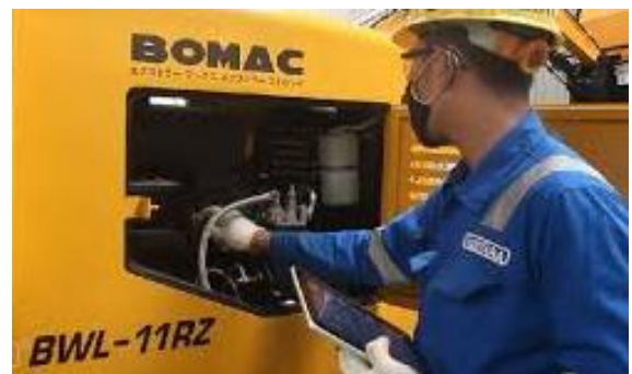
Gambar 3. Proses Pengecekan battery
